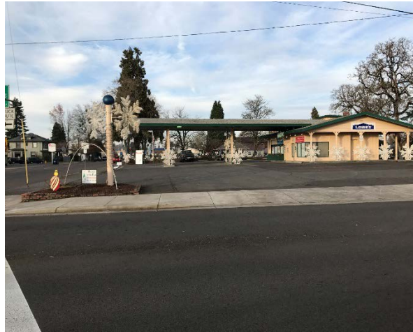
Existing Gas Station
