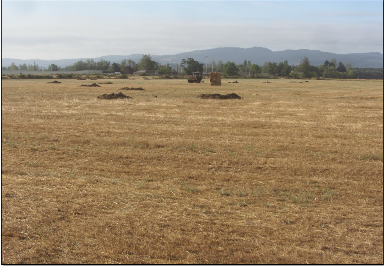
Photo 10: View of backhoe pits on north end of TL 2802 (8/14/17).
